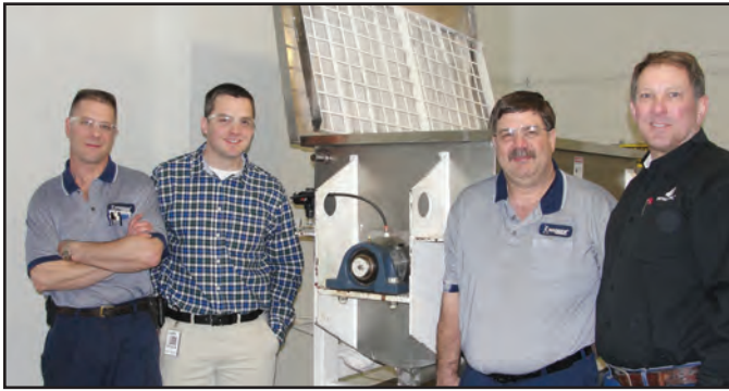
Matt Nicol (right), Inpro/Seal Regional Manager, and Neogen employees stand in front of a newly installed Inpro/Seal® Air Mizer® on one of their ribbon blenders.
